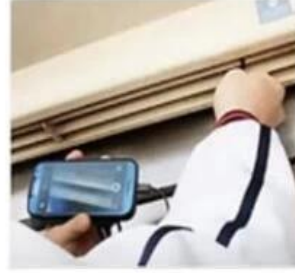
AIR CONDITIONER INSPECTION
