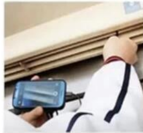
AIR CONDITIONER INSPECTION
