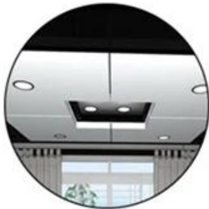
Ceiling level measurement
