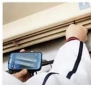
AIR CONDITIONER INSPECTION
