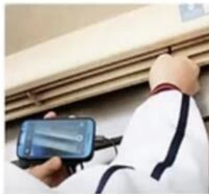
AIR CONDITIONER INSPECTION
