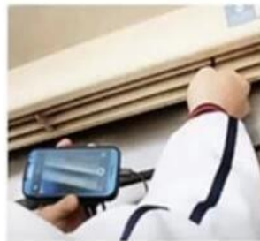
AIR CONDITIONER INSPECTION
