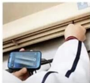
AIR CONDITIONER INSPECTION
