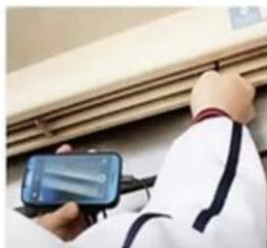
AIR CONDITIONER INSPECTION
